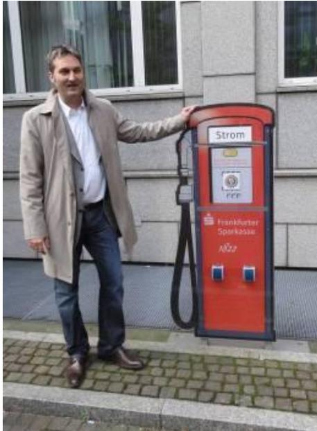
The 'Strom Tankstelle' or 'Electricity pump' is a CP installed with two dedicated EV parking places, and further two for e-bikes, on the forecourt of the Sparkasse (Savings bank) office building. They are very simple charging points, with a 220 Volt plug, designed to be highly visible to support early EV adopters. The CP draws on renewable hydro electric energy from the Main River.
